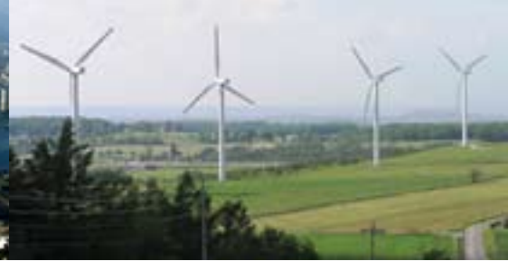
Community Energy, Inc.
